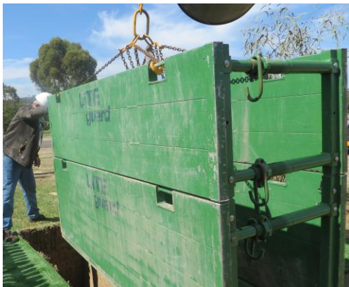
Installation of the shields
